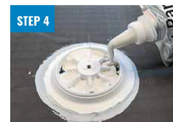
FILL WITH CHEMLINK 1-PART & PLACE CAP
