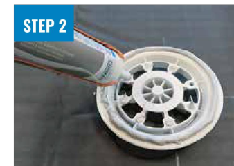
APPLY CHEMLINK M1 SEALANT
